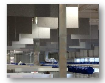
Silent Designs™ is a high performance acoustical material made from recycled cotton. This product is ideal for noise control applications. Silent Designs can be used as an acoustic wall panel or hanging baffle. Common applications are school gyms, classrooms, lunch rooms and any application where a high performance noise control product is needed. Silent Designs can help contribute to a building achieving LEED™ credits, is Class A fire rated and 100% recyclable.
