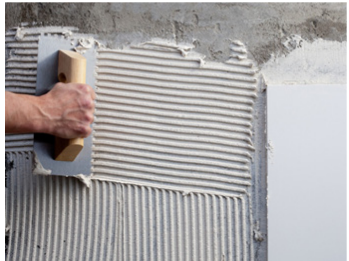
Application with trowel
