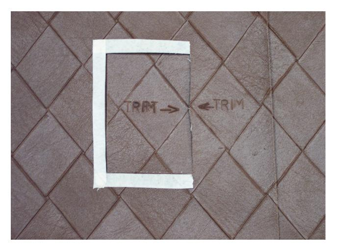
(The outlined area on the picture above has been cut out to show the trim mark on the right strip, which would normally be hidden underneath the strip on the left).
